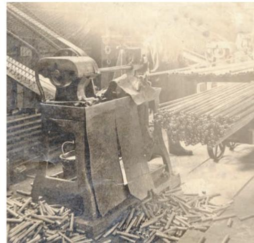
Cutting pipe into 10 foot lengths
