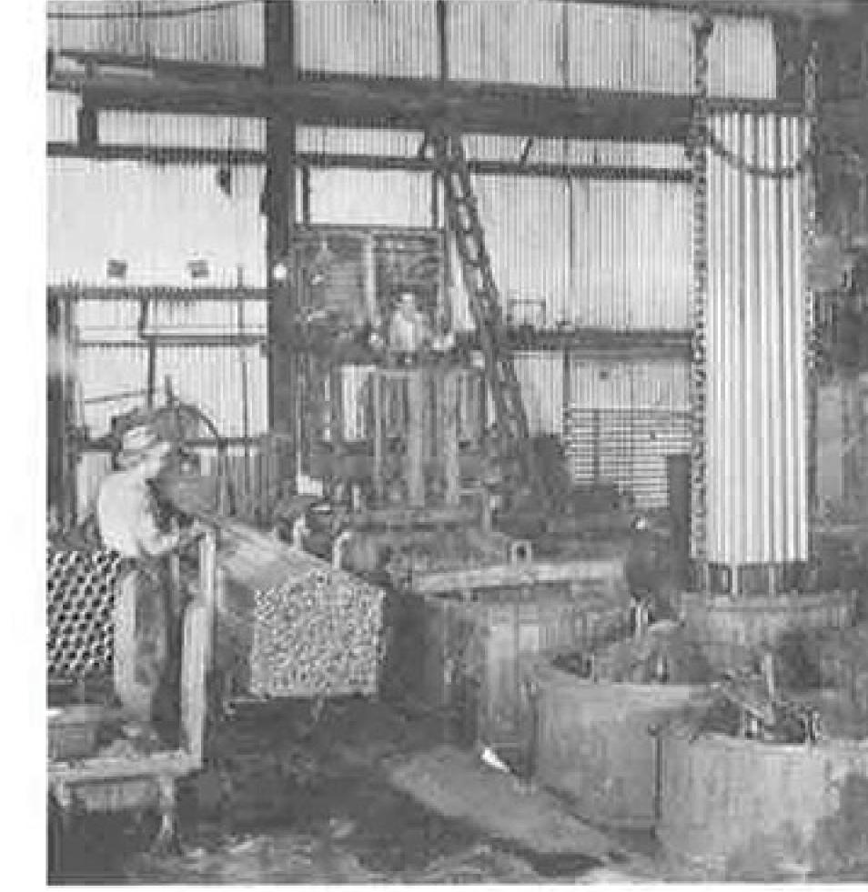
Pipe is processed through the Pickle House in this 1930's scene. Wooden tanks, 12-feet deep, were manufactured in-plant.
