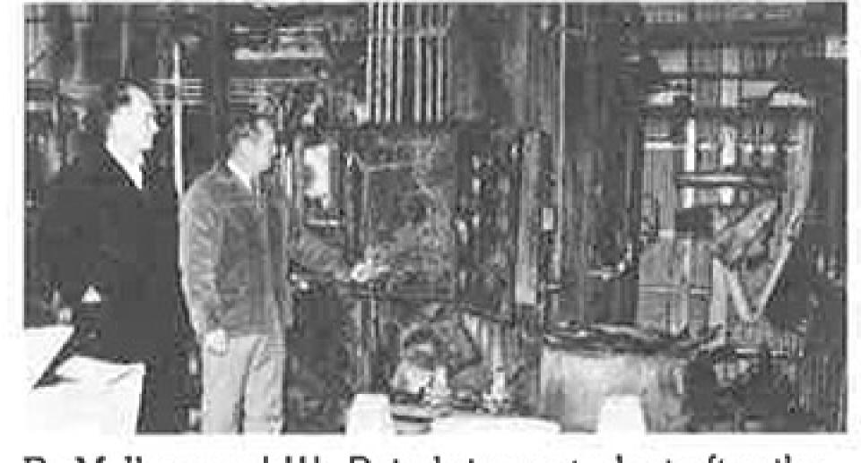
R. McIlroy and W. Beisch inspect plant after the disastrous fire of 12/30/70. Although the fire destroyed 55,000 sq. ft. of roof and knocked out all utilities, the plant was back in partial operation in 2 weeks. Much can be said for the hard work and sacrifices made by the Gilmer employees.
