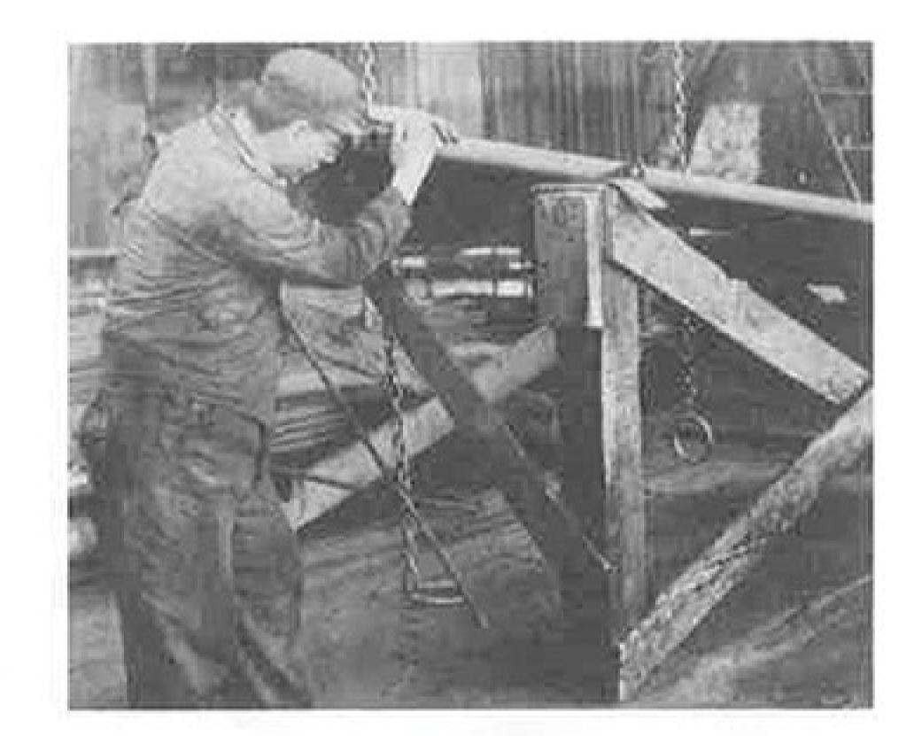
Inspector sights down the inside of conduit in a 1915 quality control procedure.
