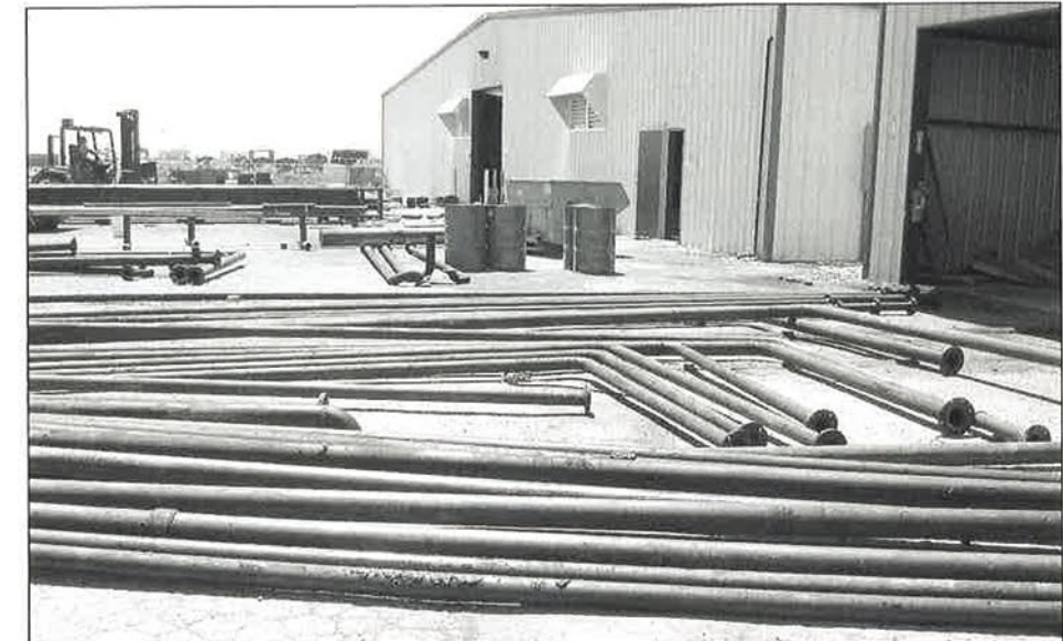
After - the pipes are cleaned, who wants to figure out how to put them back together?
