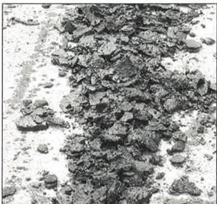
Before - this gunk was restricting the oil flow.
