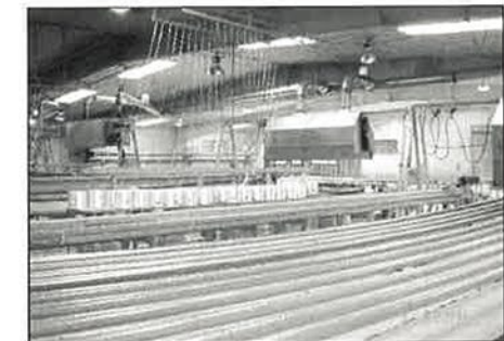
After – the new FRP facility!
