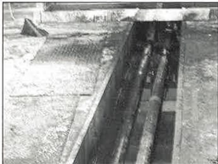
Before - all of the oil lines are almost pulled.
