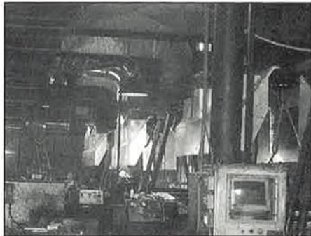
Before - the installation of hoods are just being completed.
