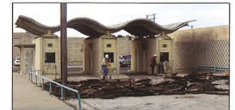
Stage One – Up comes the old asphalt.
