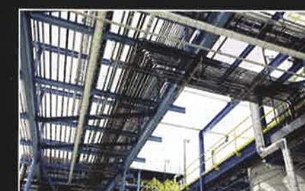
Robroy conduit installation at RT Vanderbilt Chemical.
