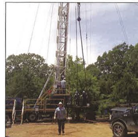
The re-run installation was located in Hainsville, Texas.
