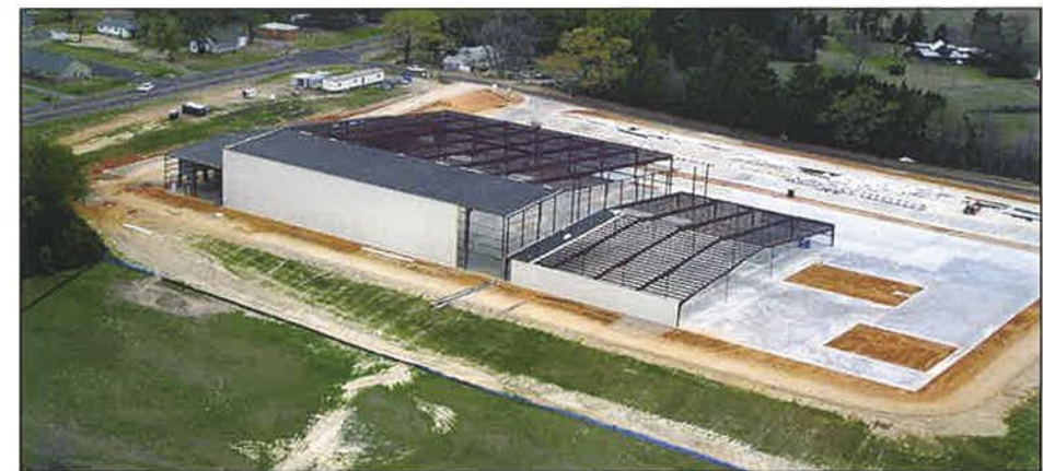
the sheeting of the exterior went up...
