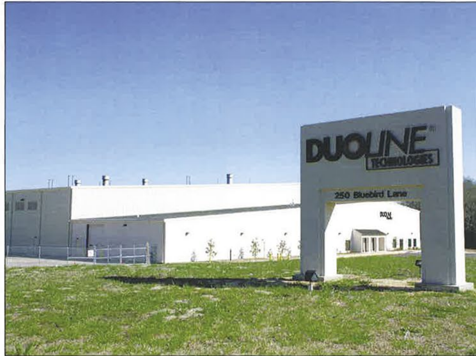
and the new Duoline facility was completed.
