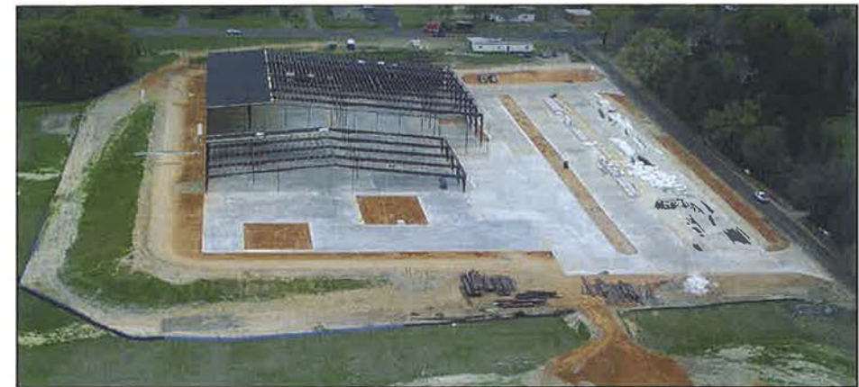
the framing of the buildings began...
