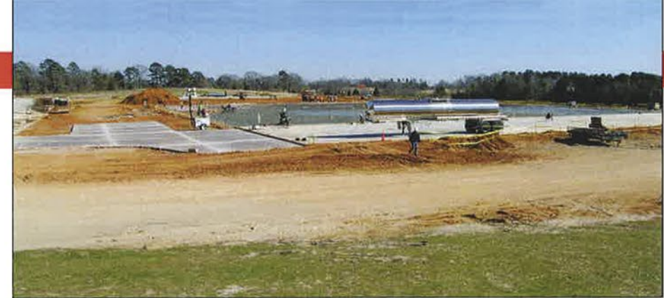
The foundation slabs were poured...
